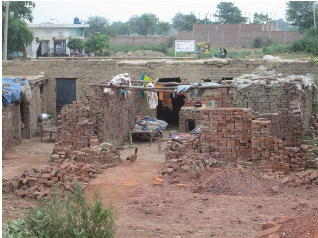
12. Workers houses, Gujrat, Pakistan. Photo by A. De Lauri
