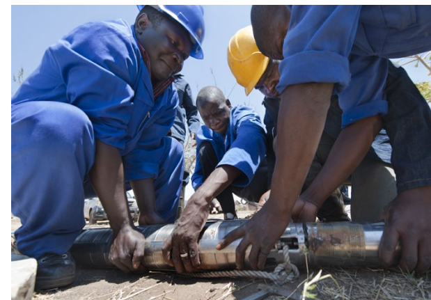
Water pipeline being repaired. PHOTO: KEN OPPRANN
