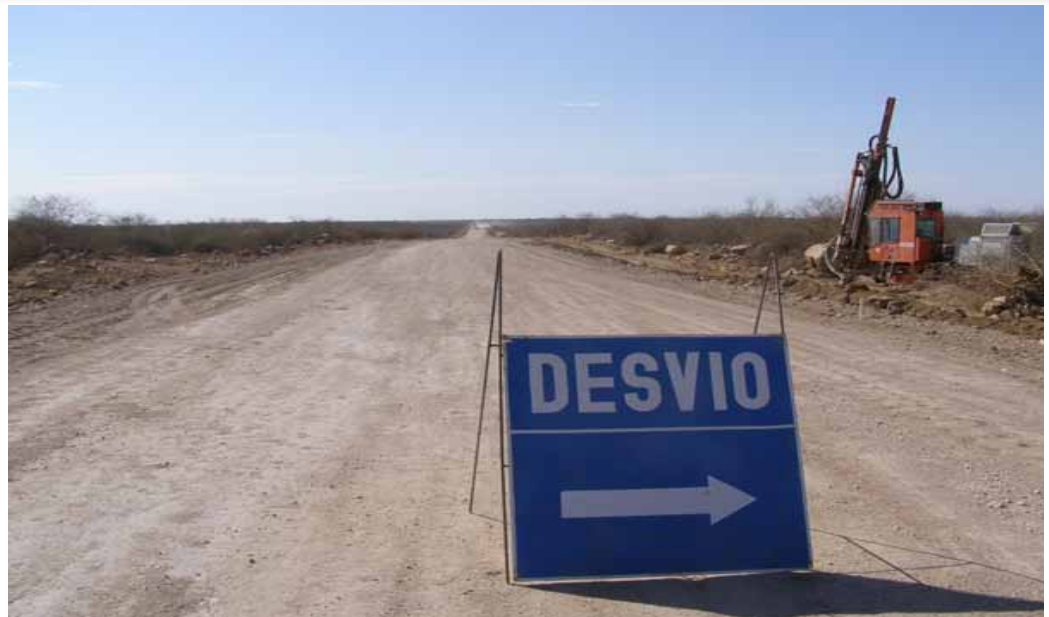
A road under construction in Angola. Photo: Aslak Orre
