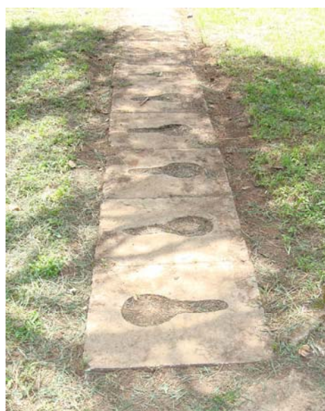
Alternative use of VIP-latrines slabs in the Maji yard, Sumbawanga
