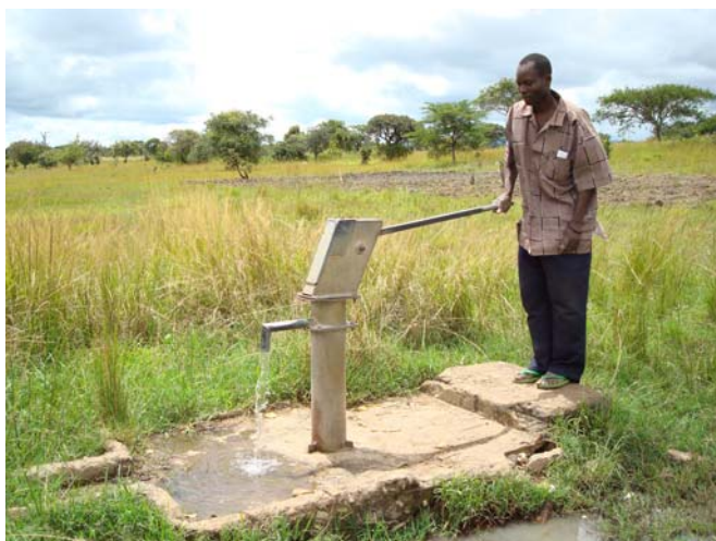
The chairman of Ntatumbila village at a borehole outside the village (the pump is the India Mark 2 type)
