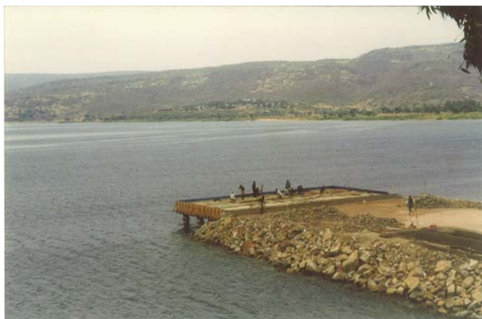
Kasanga port under construction
