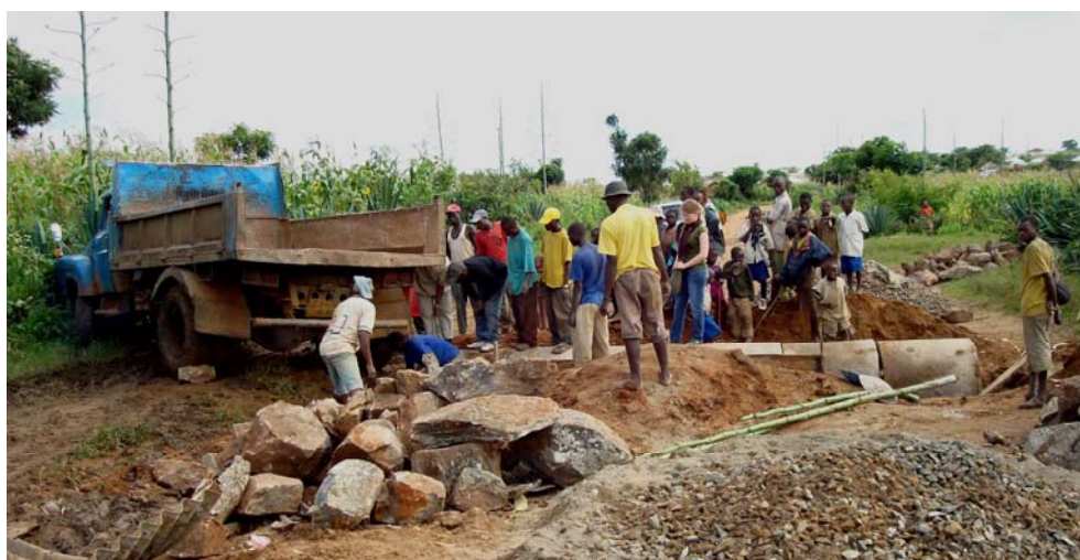
Maintenance on the Sumbawanga-Mwimbi road April 2008
