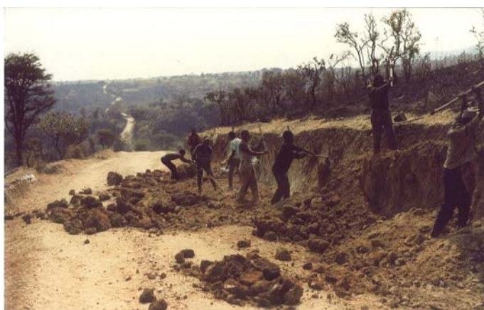
Road works on Ntendo-Muze road (1990)
