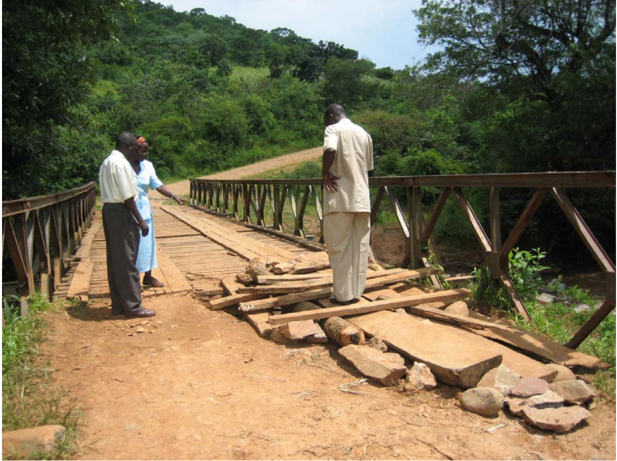
Photo 1. Poor infrastructure is one of the greatest challenges for reducing maternal deaths. In what ways do district councils cooperate with local communities to ensure that the road is passable? The picture is from Ileje DC where rain has washed away parts of a bridge (by Siri Lange)
